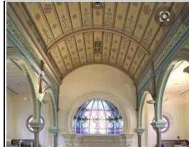
Figure 11: Decorated wooden barrel-vault ceiling in Auckland Synagogue, consecrated 1885. Photo 2018. Source: Authors.
